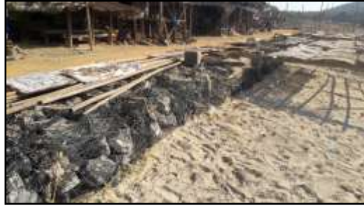
Figure 16. Seawalls in Katat-tauk Daminseik which cause changing wave refraction patterns
